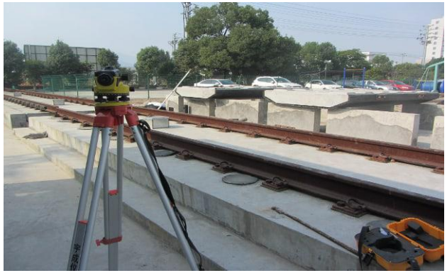
Tiantie on-site testing
