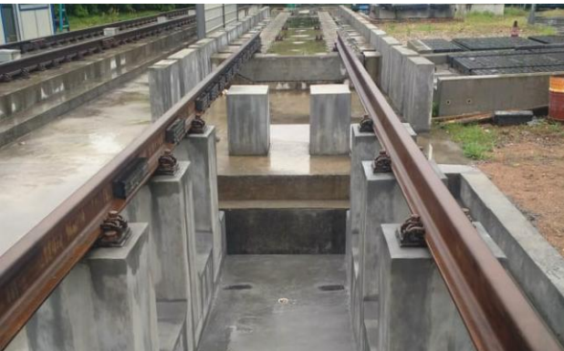
Tiantie on-site testing
