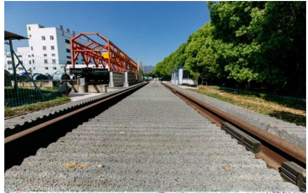
Tiantie on-site testing
