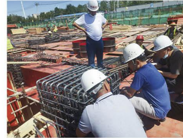
Lower buttress steel bar binding
