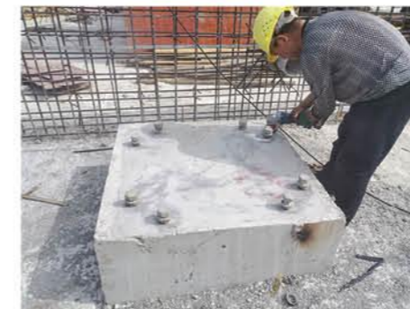
Grinding and leveling the top surface of the lower pier
