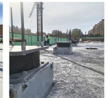
Installation of pre install compnents
