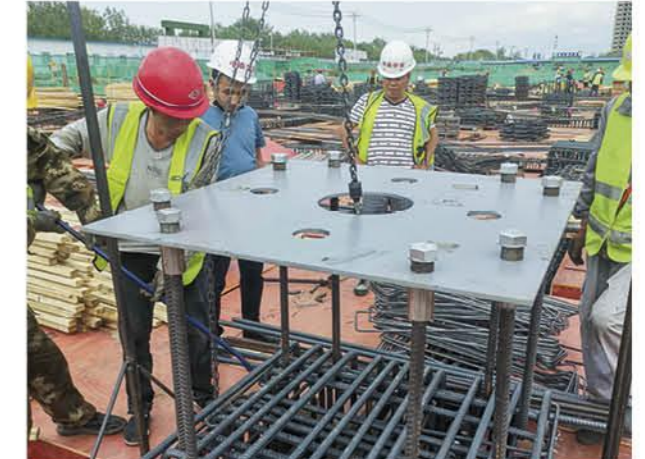
Installation of positioning plate and lower embedded components
