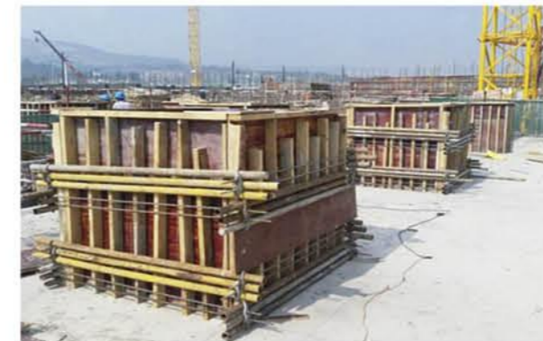
Lower pier formwork support protection
